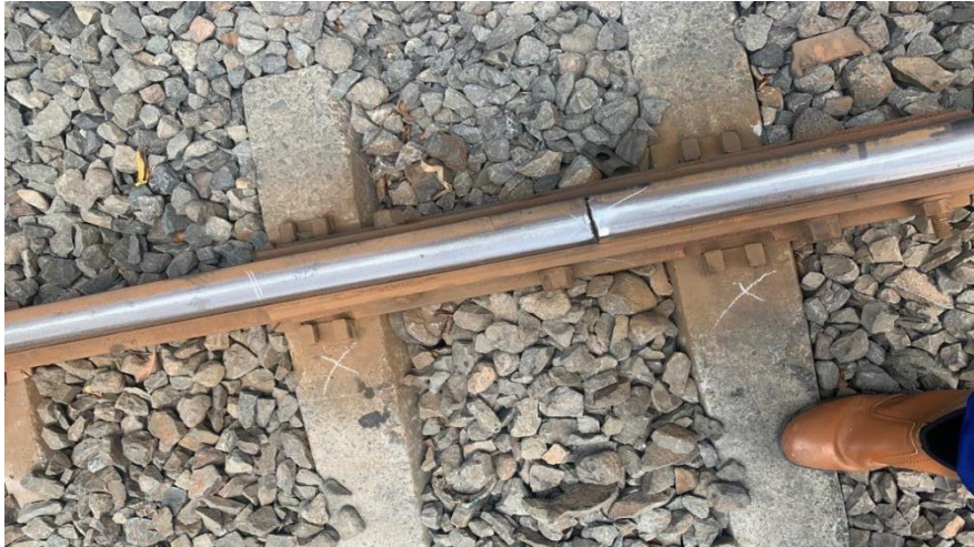
Figure 5 Missing Anchor
