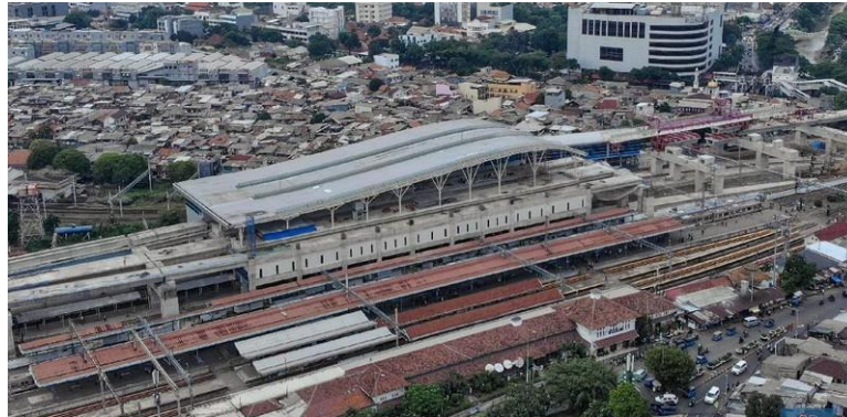
Fig. 1: Double-Double Track Project
