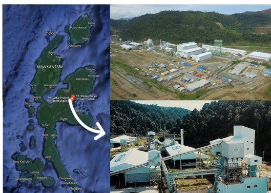
Figure 4. Remote area project location at Halmahera, North Maluku
